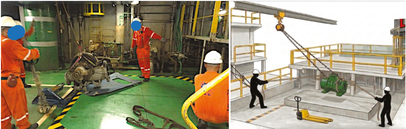
Figure 3 System with hoists and cables for mounting a pump on a pallet jack
