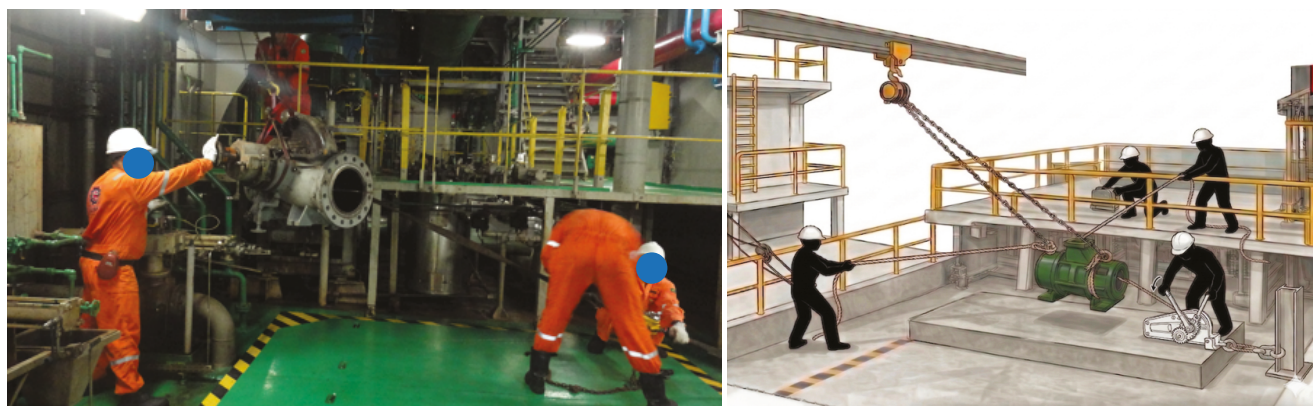
Figure 2 Operators pull the pump with the winch to navigate around obstacles
