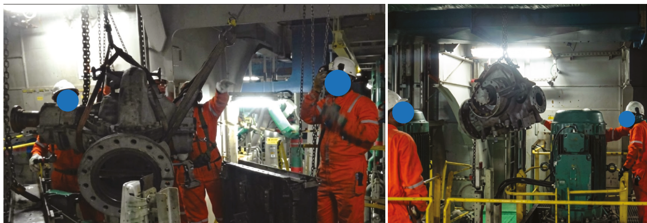
Figure 1 Lifting, removal of the pump from the cradle, and alignment with the monorail
